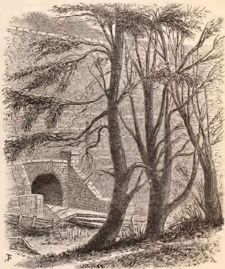
CROTON AQUEDUCT BRIDGE ACROSS THE POCANTICO.
