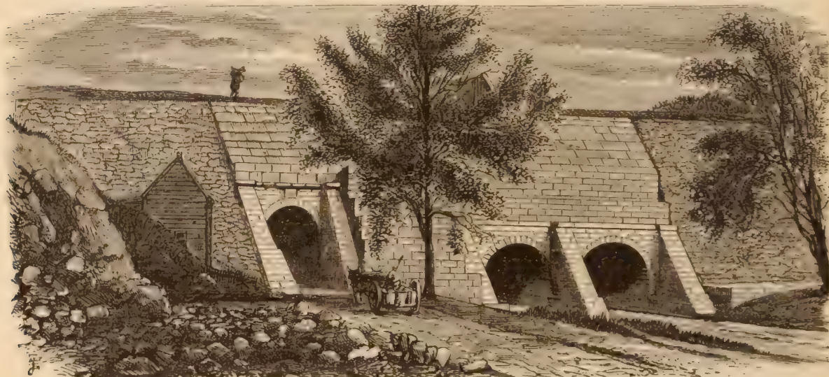
AQUEDUCT BRIDGE OVER SAW-MILL RIVER, AT YONKERS.
